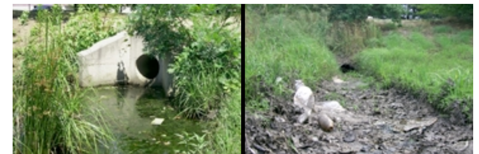
Improper maintenance can quickly lead to a malfunctioning, smelly and unsightly basin that could be a health hazard.
