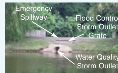
Retention Basin Outlet. An outlet pipe may also release water mid-depth; water at that level is assumed to have longer residence time and be cleaner than surface water.
