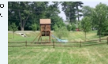
Detention basins can be used for recreation. This basin makes up a backyard. A playset and fence have been installed. However, these basins temporarily fill with water. Nothing inside the basin should impede water flow or block an outlet.
