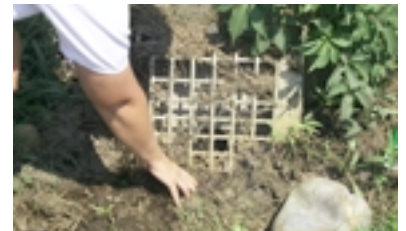
Simply clearing the outlet opening can help prevent a detention basin from clogging and failing to function.
